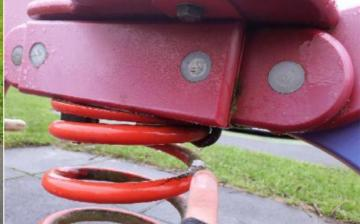
Finding: The spring clamps are loose Action: Tighten all loose fixings
