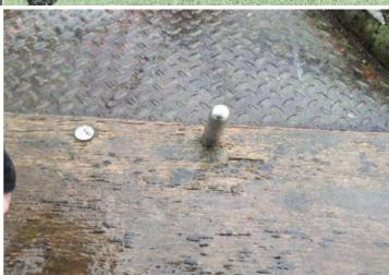
**Finding:** There is/are finger entrapment/s in the platform due to missing fixings and the item fails to meet the requirements of BS EN 1176 Part 1 4.2.7.6 Entrapment of fingers
